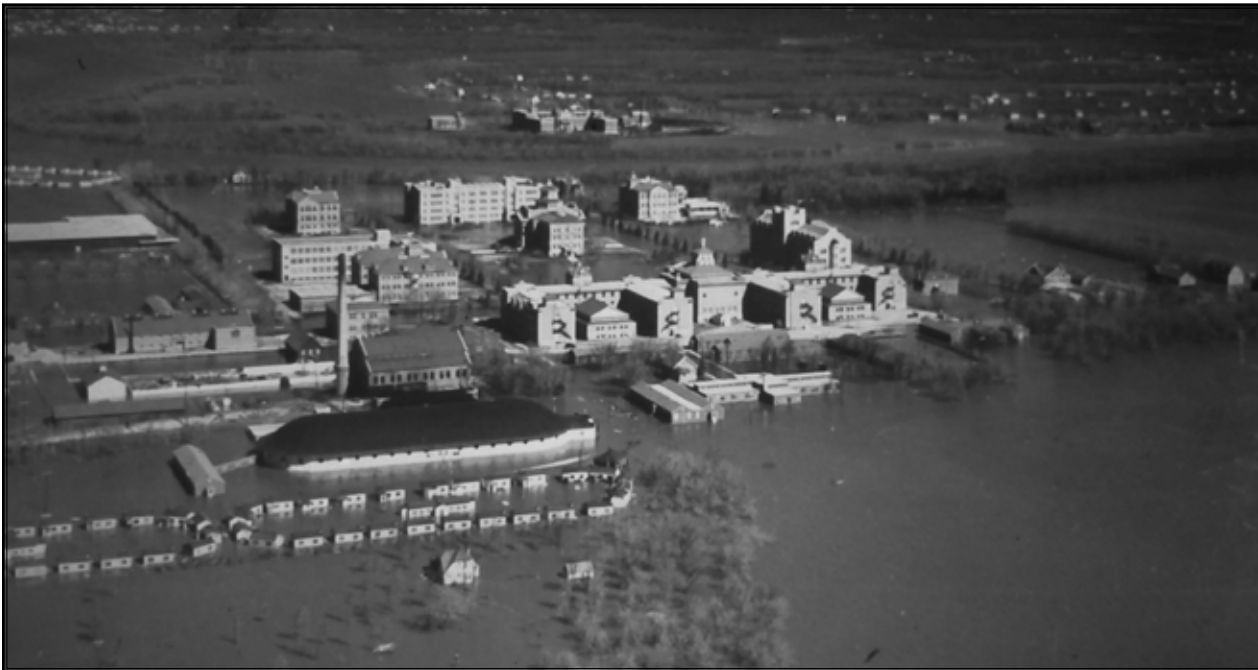
■ The Veterans' Villages and the wartime huts behind the Manitoba Union Building seen during the 1950 Flood.
