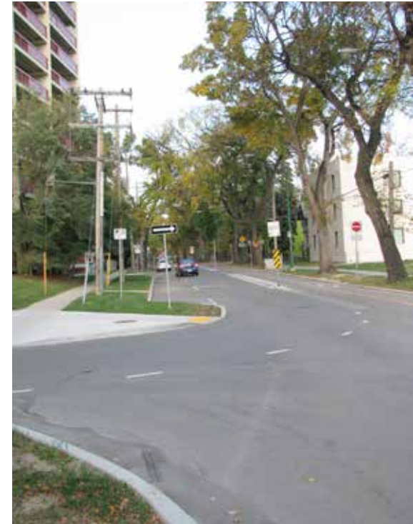
Figure 14: Curb extension: An extension or bump-out of the curb used to reduce the roadway width. Can be used at pedestrian crossings to narrow the distance pedestrians need to cross and slow motor vehicles.
