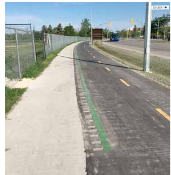
Figure 10: Typical 4.5 m wide multi-use pathway with separation of pedestrian and cyclist users. Pedestrian path 1.5 m concrete. Bike path 3.0 m asphalt
