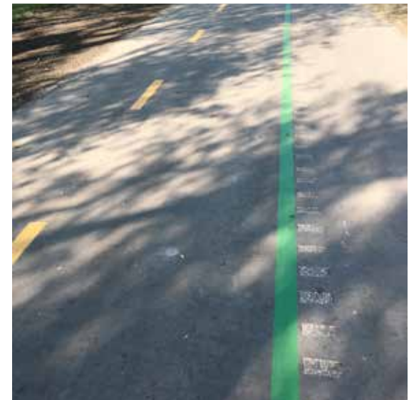
Figure 20: Multi-use pathway on Markham Road with separation between pedestrians and cyclists.
