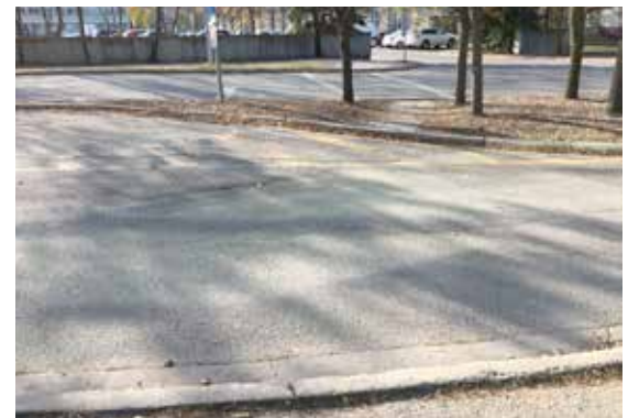
Figure 18: Example of a gap in accessible connectivity in the pedestrian network where curb ramps do not exist for an existing crossing.
