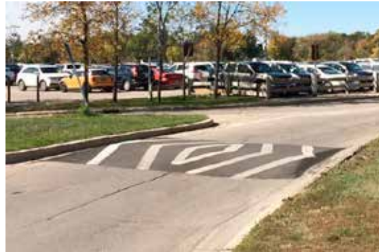
Figure 12: Speed Hump: Vertical deflection in the roadway used to slow motor vehicle speeds.
