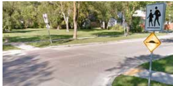
Figure 13: Raised crosswalks are crosswalks above the level of the street at the point of a crossing. They are outfitted with crosswalk markings and signage to channel pedestrian crossings, providing pedestrians with a level street crossing. They can be used as traffic calming in a similar way as speed humps. Raised crosswalks increase safety for pedestrians by increasing their visibility at the crosswalk as well as slowing motor vehicles down at the crosswalk.
