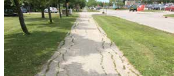
Figure 16: Examples of deteriorating surface condition on asphalt multi-use pathways.
