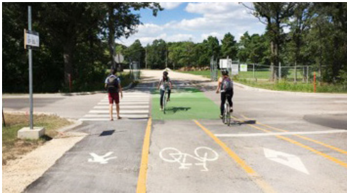
Upgraded pedestrian and cycling infrastructure
