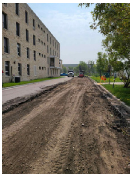
Laneway asphalt road construction
