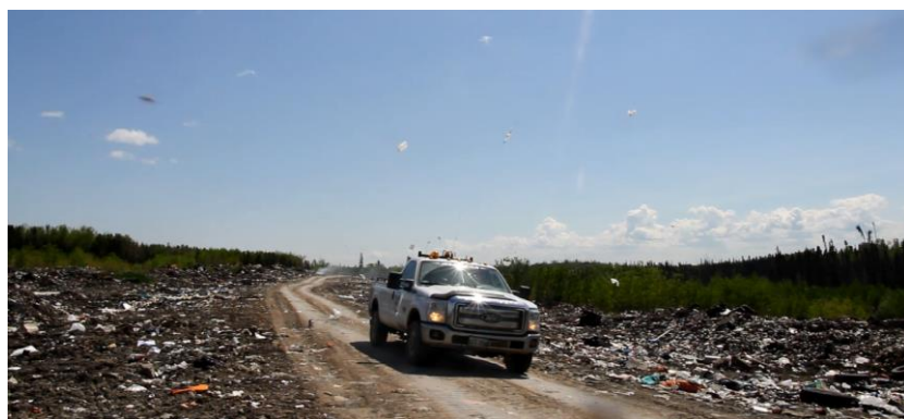
Figure 2: Road passes on top of garbage dump where community members typically dumped wastes. Waste materials were not compacted and can be seen flying around the communities.
