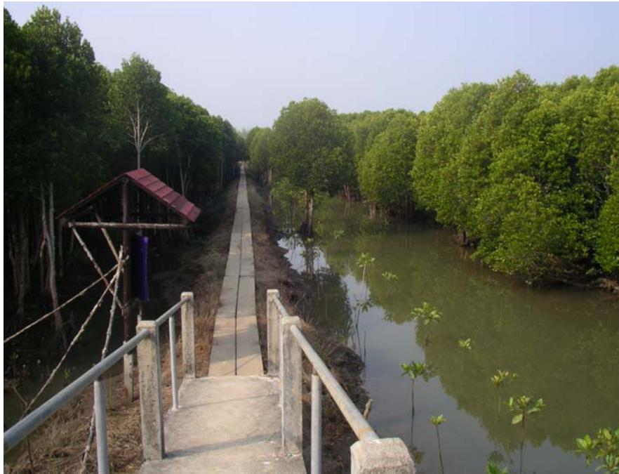
Plate 3: A portion of the walkway through the mangroves. Pred Nai constructed the walkway with funding from the Social Investment Fund.
