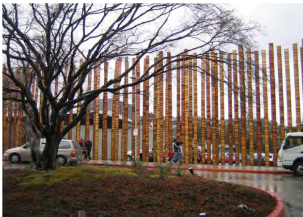
Concealing servicing areas
