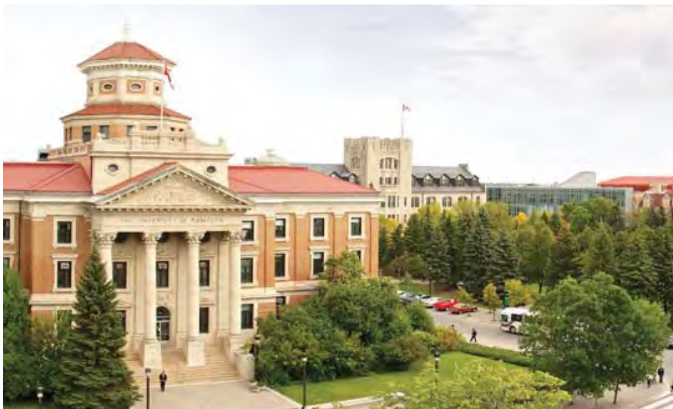
Panoramic view of Administration Building
