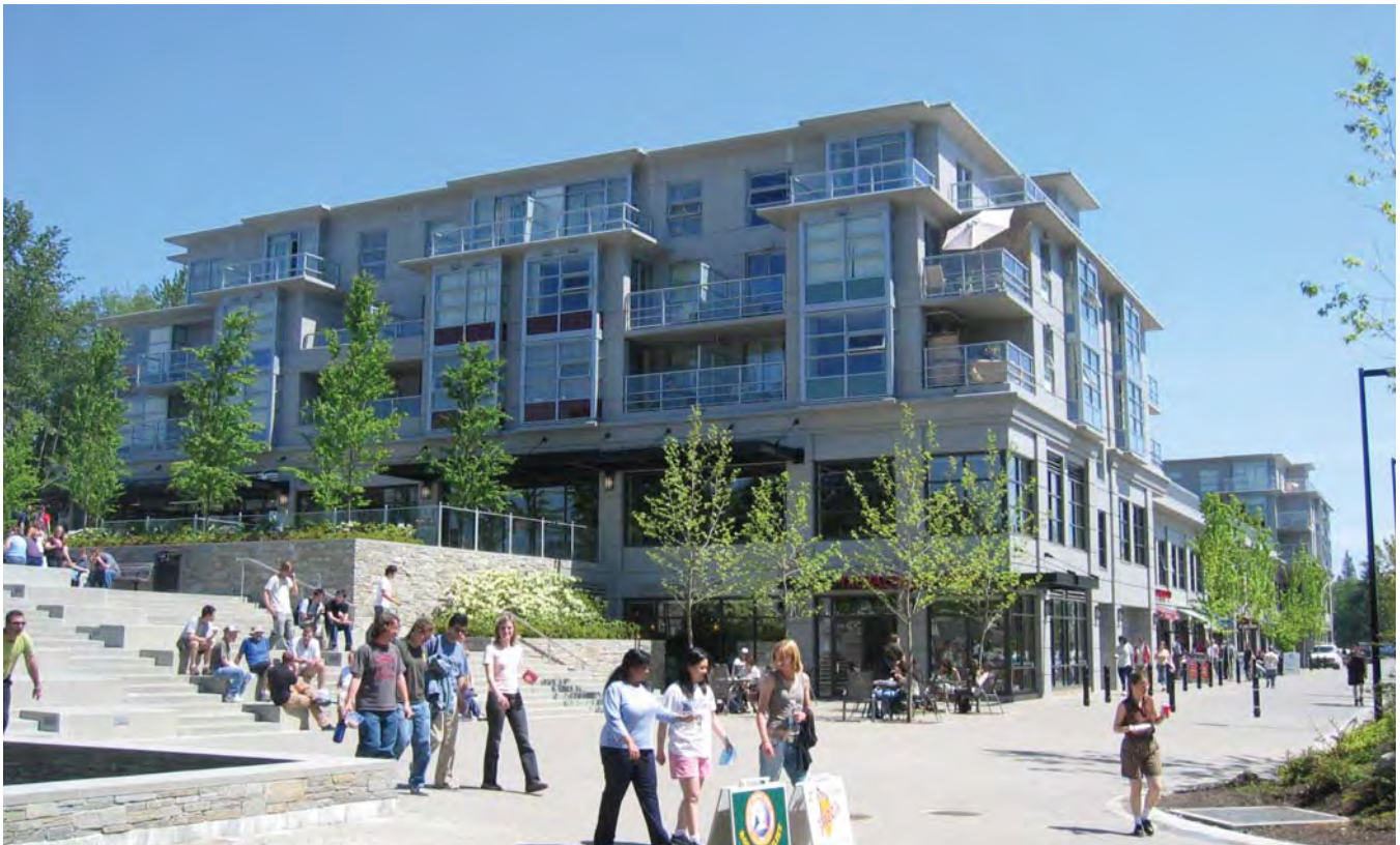
A successful built form framework seamlessly integrates and animates all aspects of the public realm
