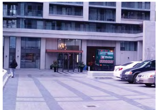
Internal servicing area with low-profile access
