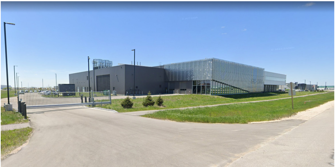
Figure 4: Active transportation path along the National Research Council of Canada on Red Fife Roadw
