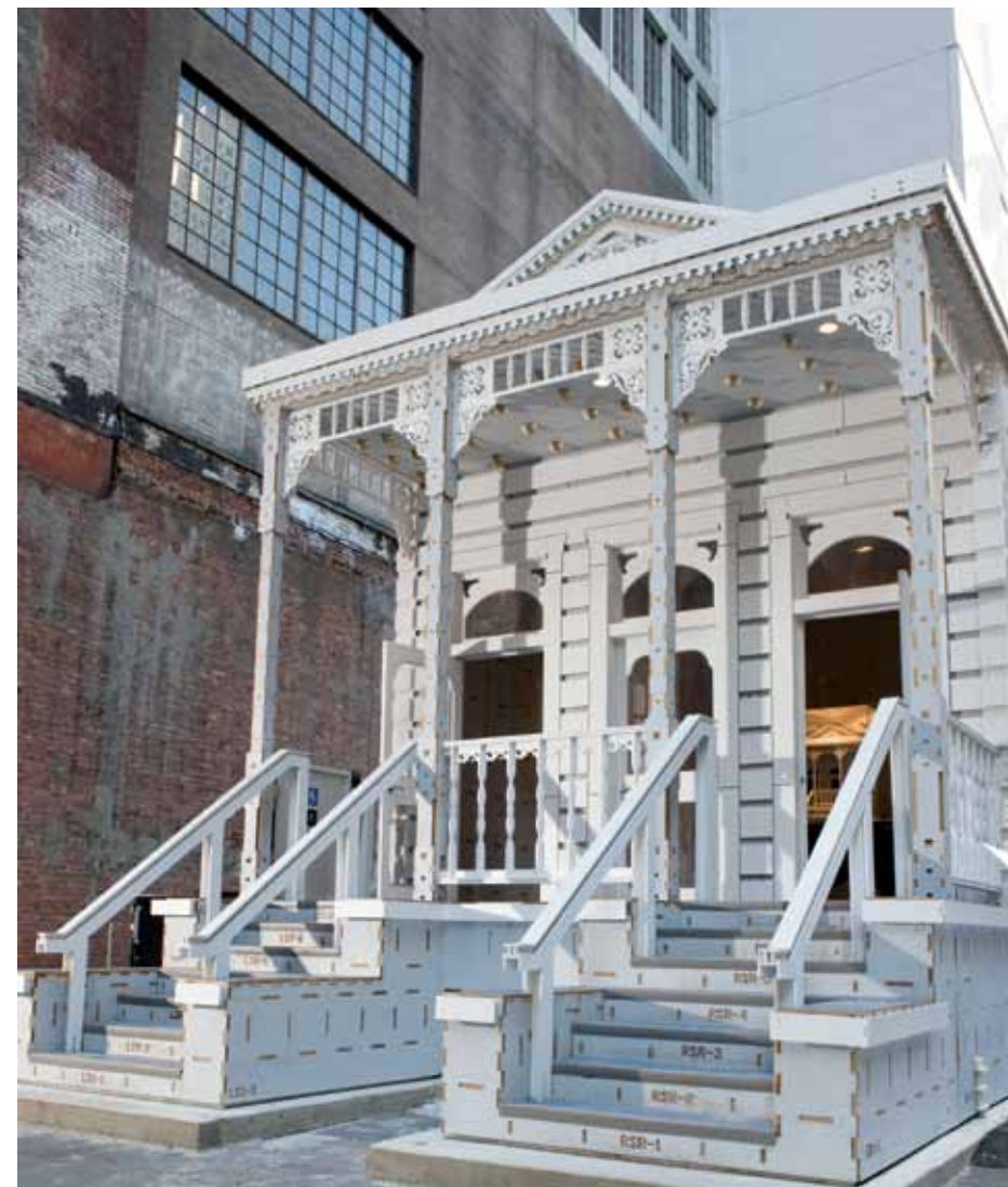
Left: "Housing for New Orleans" by Lawrence Sass. A digitally fabricated house that can be assembled using a rubber mallet. Images courtesy of Lawrence Sass.
