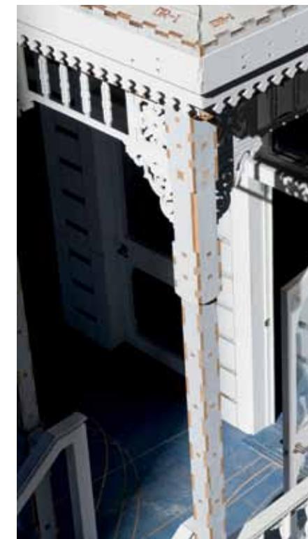
Left: "Housing for New Orleans" by Lawrence Sass. A digitally fabricated house that can be assembled using a rubber mallet. Images courtesy of Lawrence Sass.
