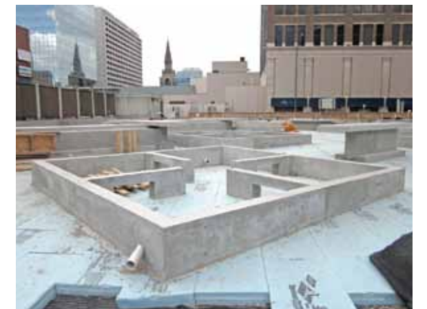
Millennium Library tree vaults under construction. The vaults will facilitate removal and re-use of mature trees when the new roof membrane is replaced decades from now
