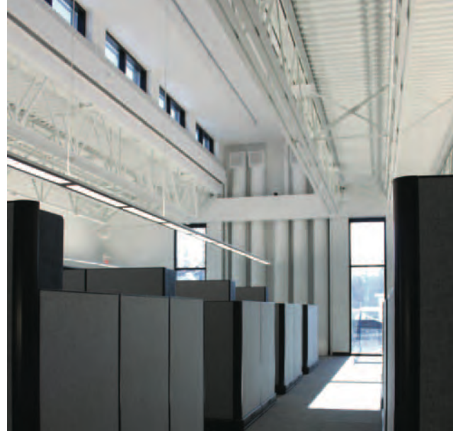
Interior offices with view of the armatures that carry the building's mechanical systems and host the clerestory windows.
