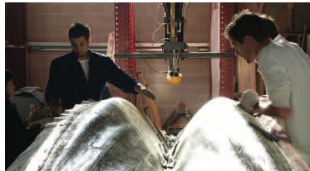
Students constructing a thin-shell structural vault on a fabric-formed mold.
