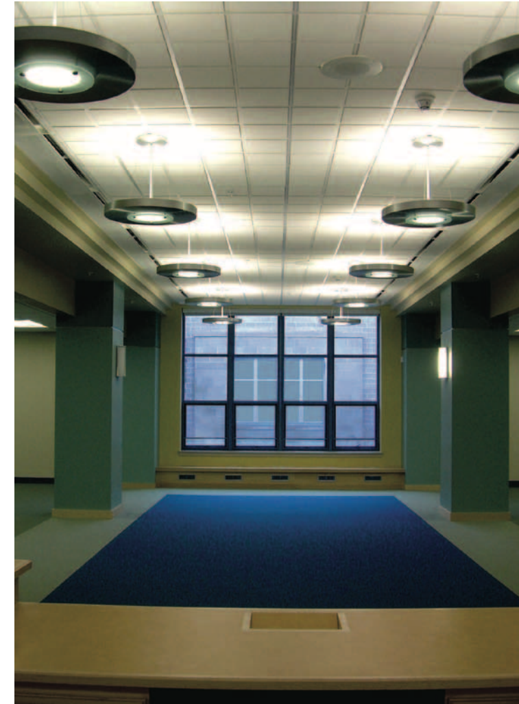
Price Chilled Beams in an architectural ceiling
