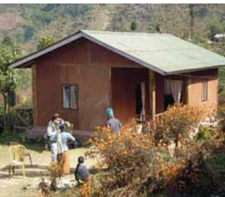
The all-bamboo model house (left). Corrugated bamboo roofing sheets (CBRS) were found to delaminate – the Bamboo for Habitat Micro-Enterprise has since corrected the design to allow for fabrication. The homeowner has developed a bamboo furnishings business (right).
