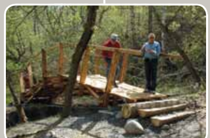
construction of the arched-truss bridge over an existing ravine along the Clearwater Nature Trail
