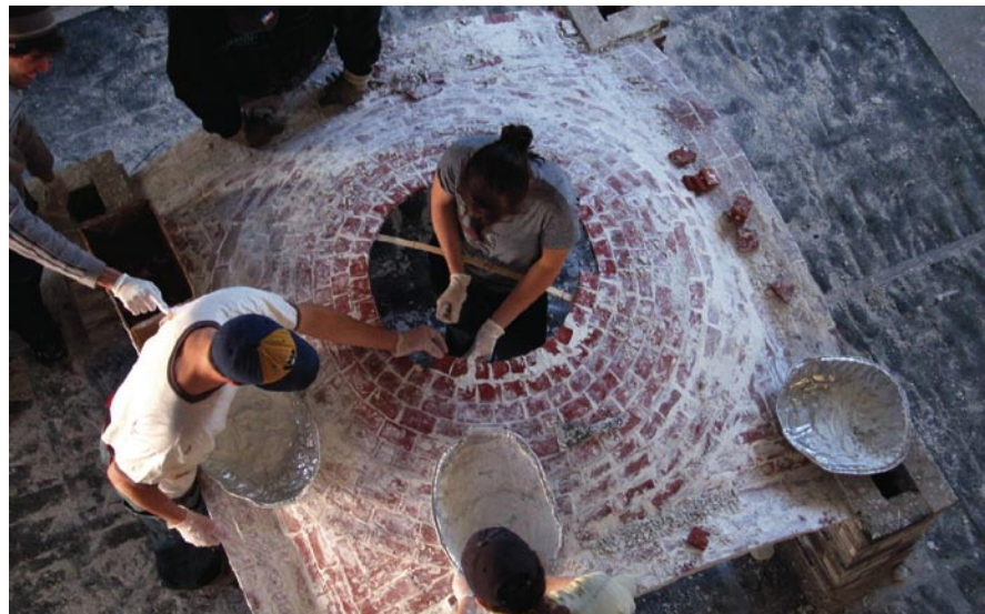
finishing the oculus on the 2006-2007 dome
