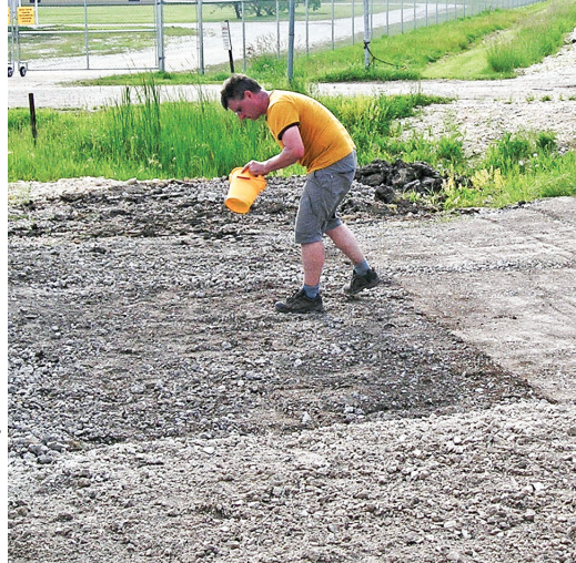
Sowing before and after roller compaction
