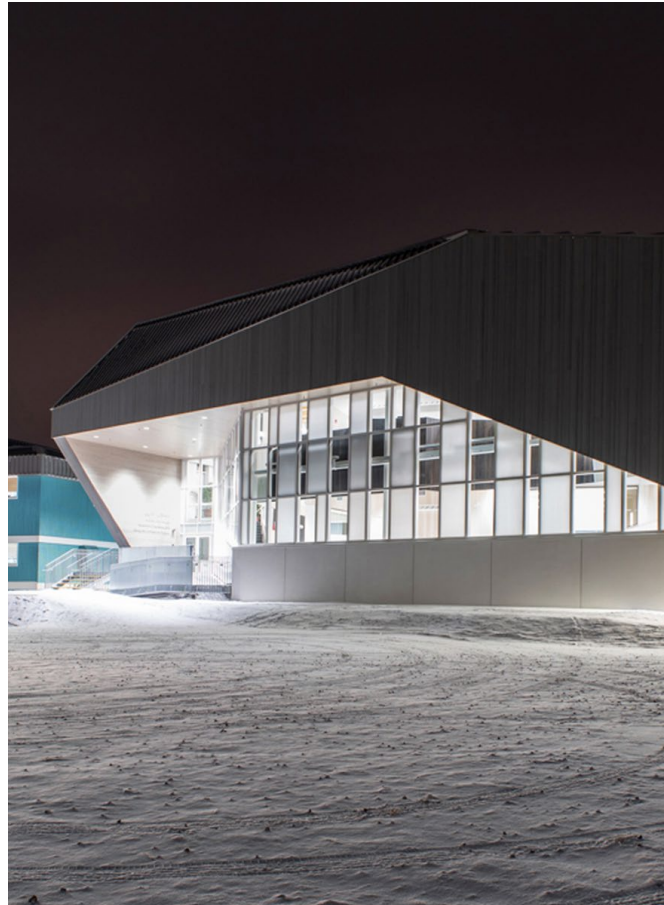
Photograph by Julie Jira. Nunavut Arctic College Expansion & New Community Learning Centre, Cibinel Architecture Ltd., 2019.
