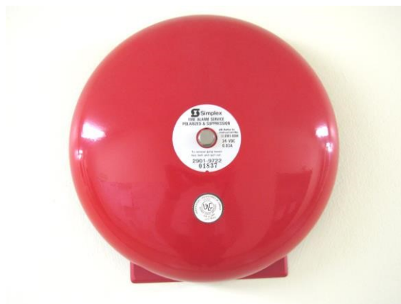
Fire Alarm Bell
