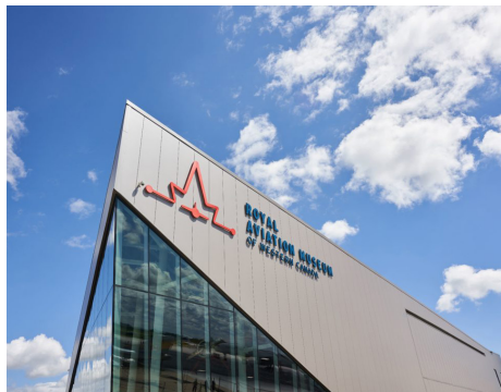
Exterior of museum. David Lipnowski photo
