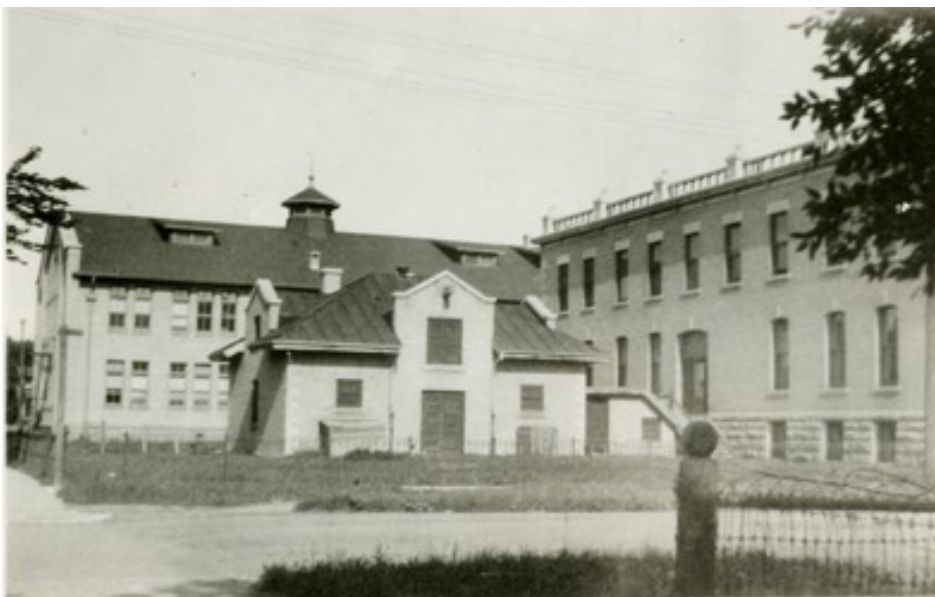
1. The Coach House at Bannatyne Campus was intended for the Dean of Medicine to park his horse-drawn sleigh, 1924. Faculty of Medicine Archives, Medical Campus Architecture collection, UMFMA 004.
