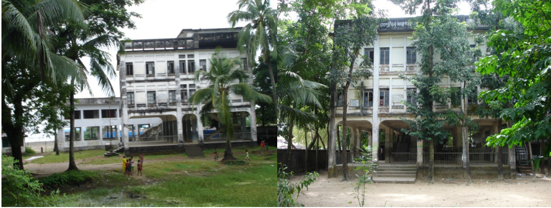
Pictures 15 and 16: Cyclone shelters in the Cox's Bazar area.
