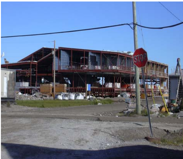
New quad-plex construction – social housing
