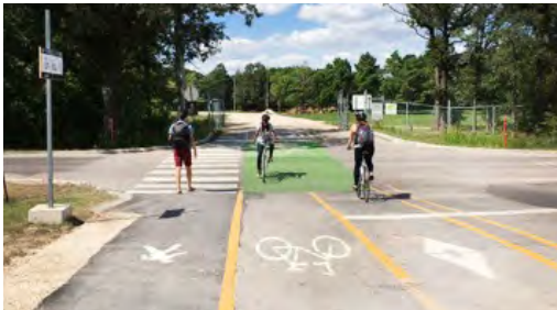
Upgraded pedestrian and cycling infrastructure
