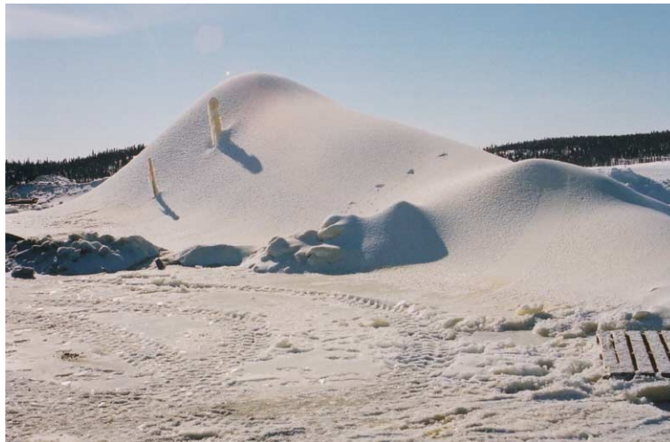
Fig. 2. Spray ice mound after completion.
