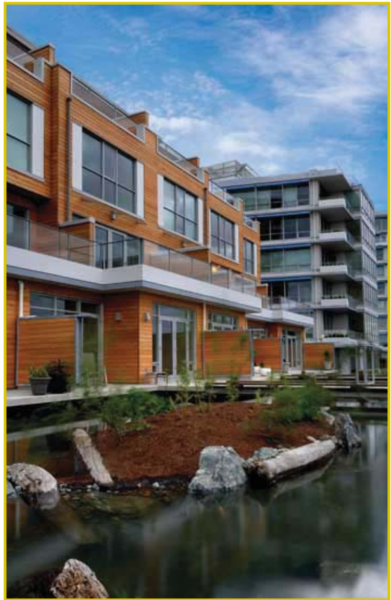
Completed townhouses and high-rise condos in Dockside Green
