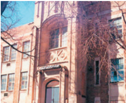
Remnants of the Gathercole Building, now demolished, will be used in the River Landing Project. (Image: www.riverlanding.ca )
