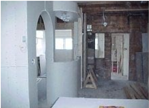
HOP house during renovation
