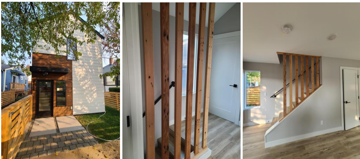
Images from a new build by Sledge in Seattle where salvaged lumber was used for finishing, both inside and outside of the house.
