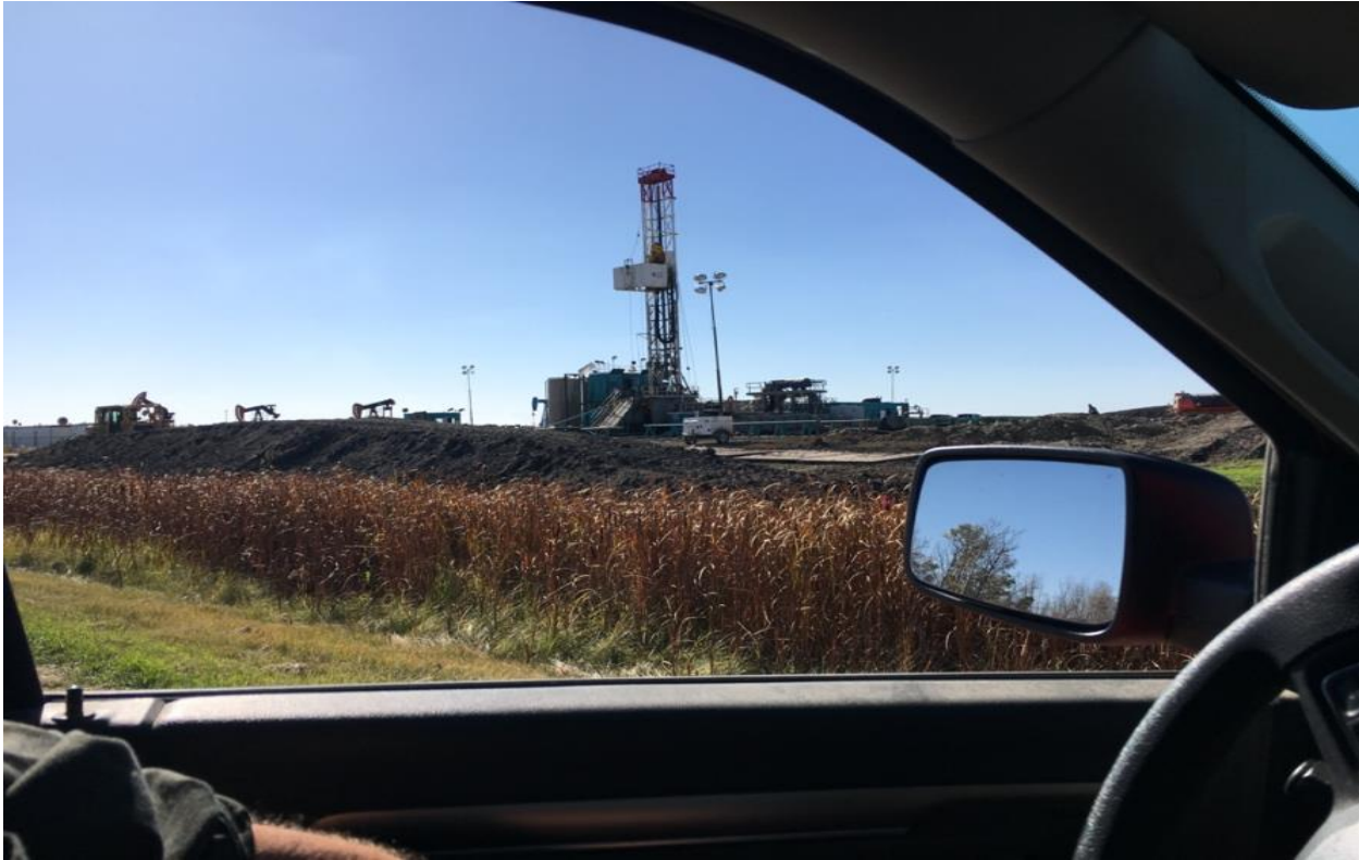
Figure 9: Drilling operation, Manitoba
