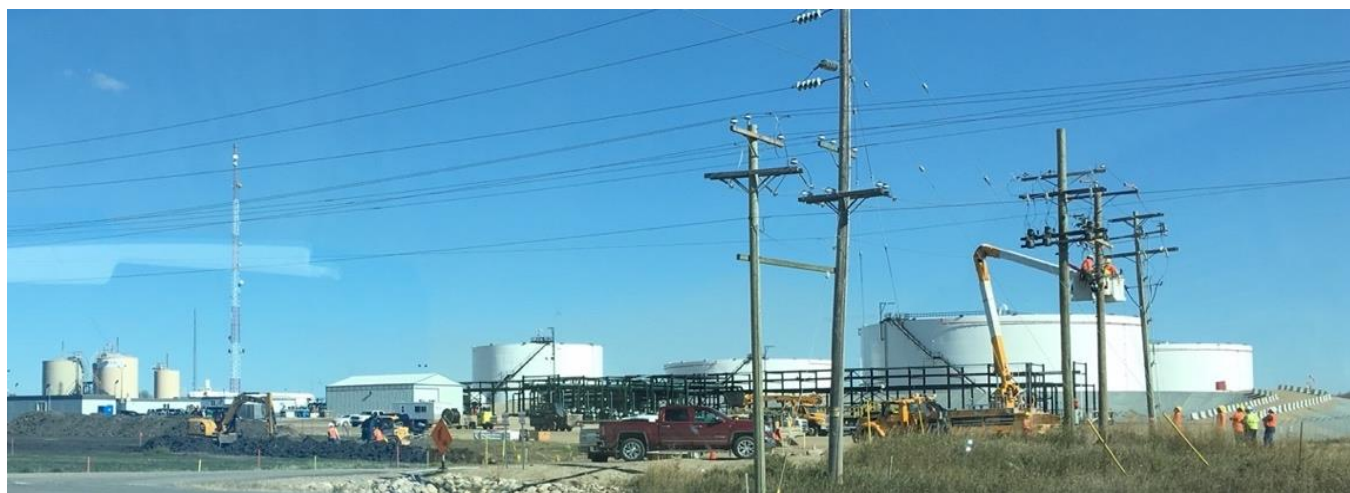
Figure 16: Tundra Market Limited Holding Facility, Manitoba
