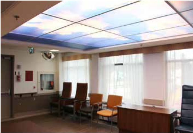
Circadian lighting was added to dining rooms to better match natural lighting throughout the day.
