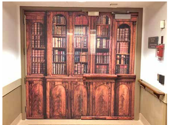
The bookcase film placed on the exit door is one of the changes made during the renovation.
