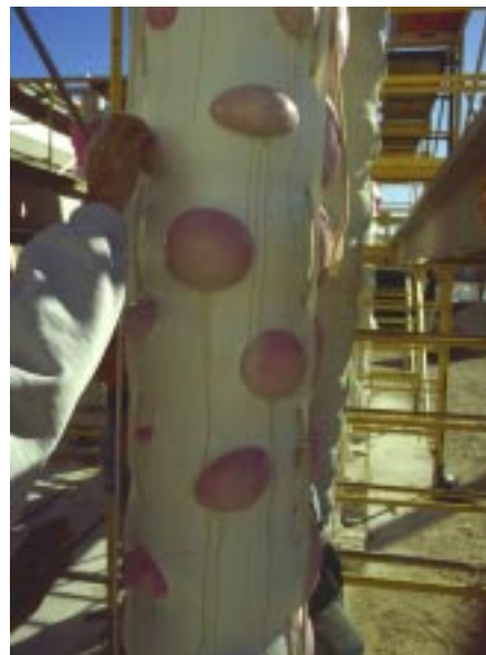
12. Formwork for the precast column shown in fig. 11. A 'spandex' liner is allowed to deflect through openings in non-stretch liner.
