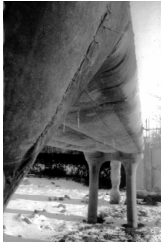
Figure 7. Photograph from below of one-way slab with integral beams and columns.
