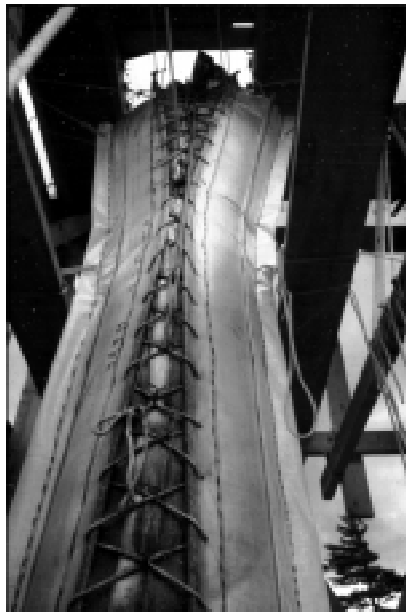
Figure 1. Woven polyethylene column formwork filled with concrete.
