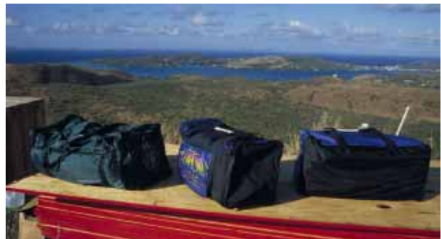
Figure 2. Lightweight fabric formwork for 13 individually dimensioned and detailed columns were shipped by air to Culebra, PR in three small duffle bags.
