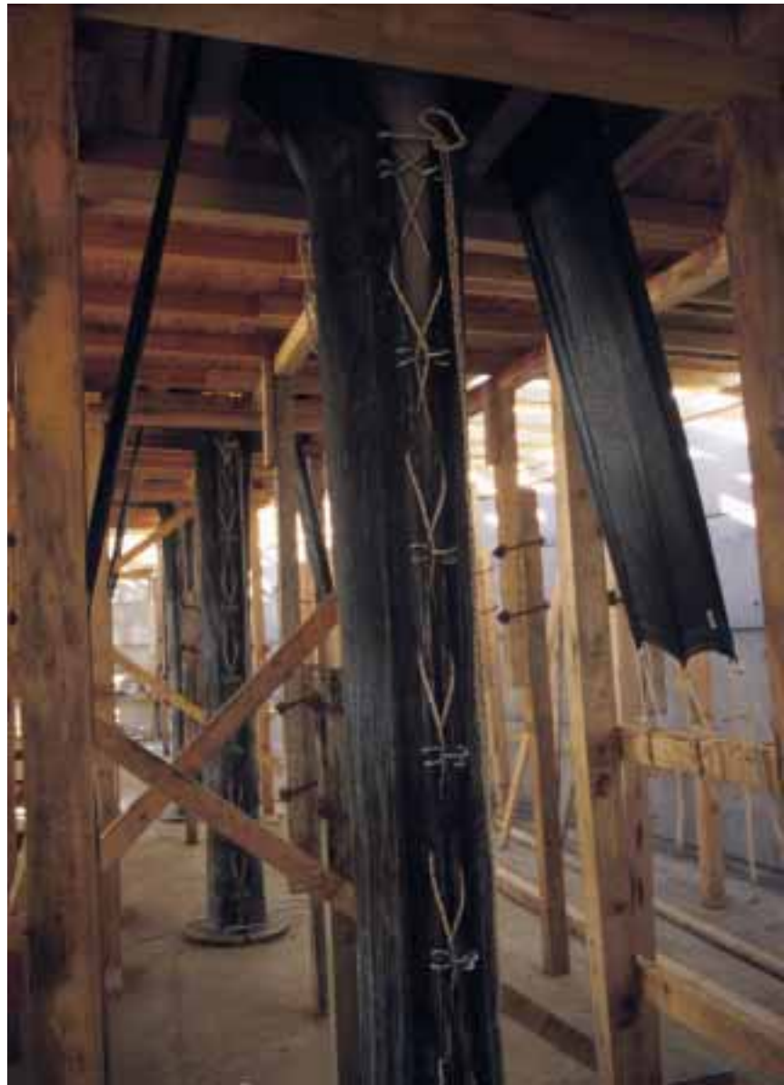
Fig. 1. Fabric columns formworks awaiting concrete placement
