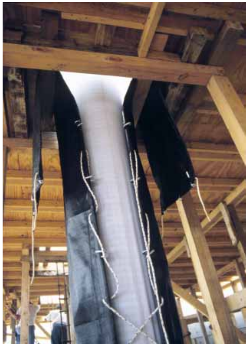
Fig. 4. Inner liner with outer jacket, prior to jacket lacing and pre-tensioning.
