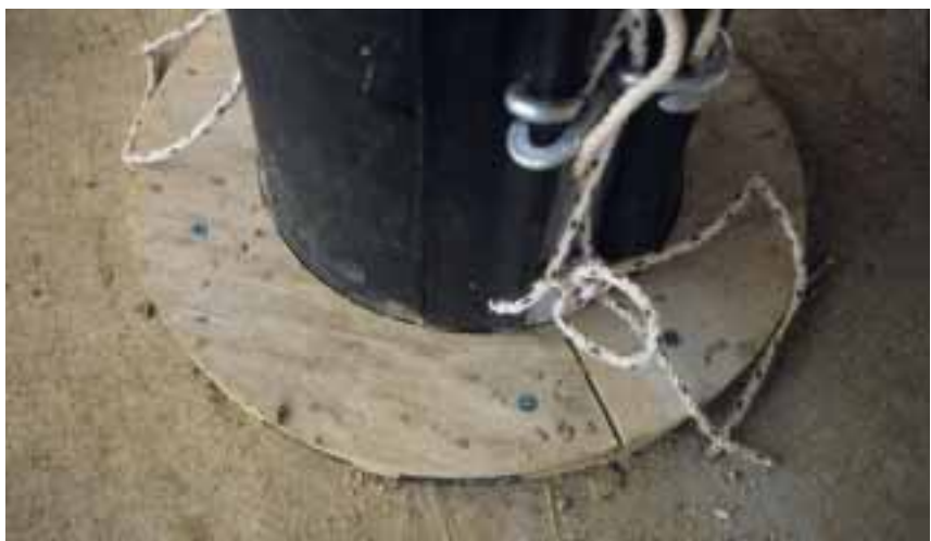
Fig. 5. Bottom of fabric formwork attached to floor slab
