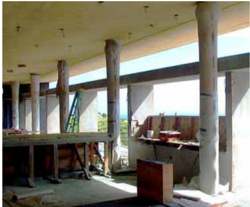
Fig. 10. View of Casa Dent interior under construction.
