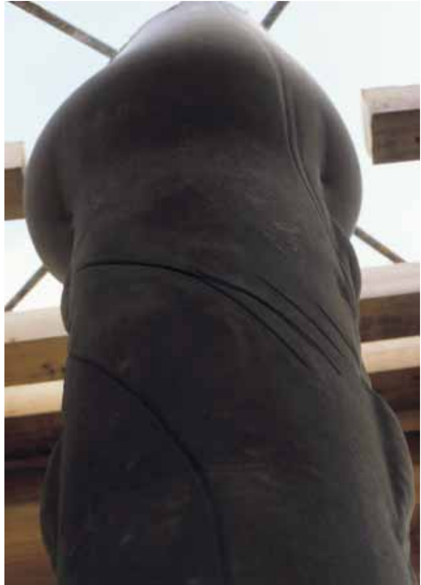
Fig. 8. Column capital showing the impressions left by the torsion or the inner stretch liner, and the fine surface finish obtained by the filtering action of fabric formworks.
