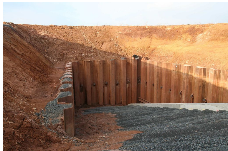
FIGURE 11 | Sheet pile wall in a building foundation
