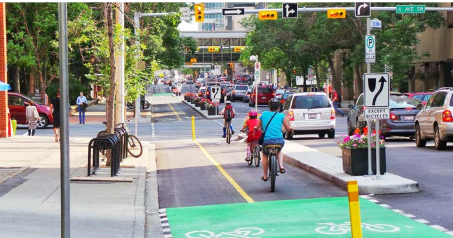
Above: 7 St S.W and 3 Ave S.W. Cycle Track received from The City of Calgary
