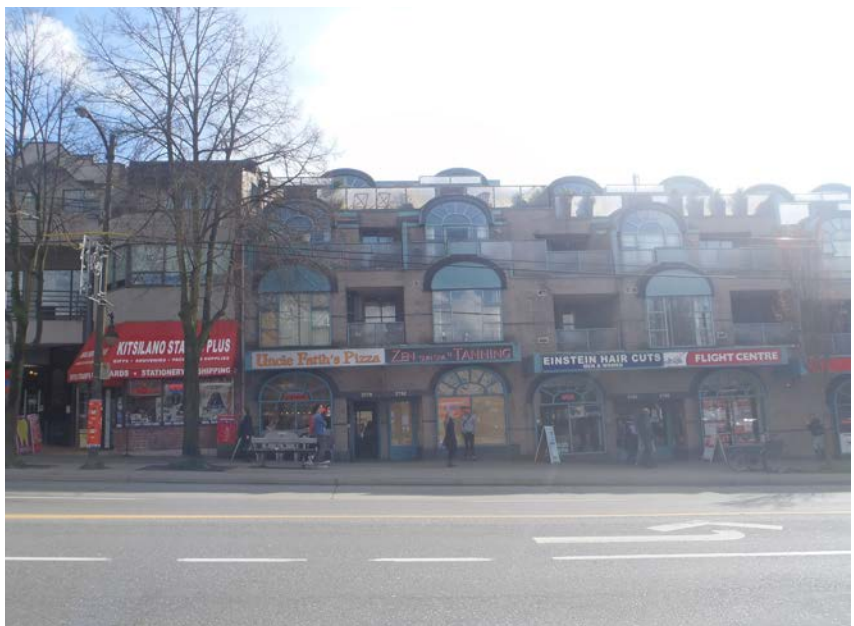
West Broadway street frontage with a mixture of outright and conditionally permitted uses (Source: Madeleine Koch)
