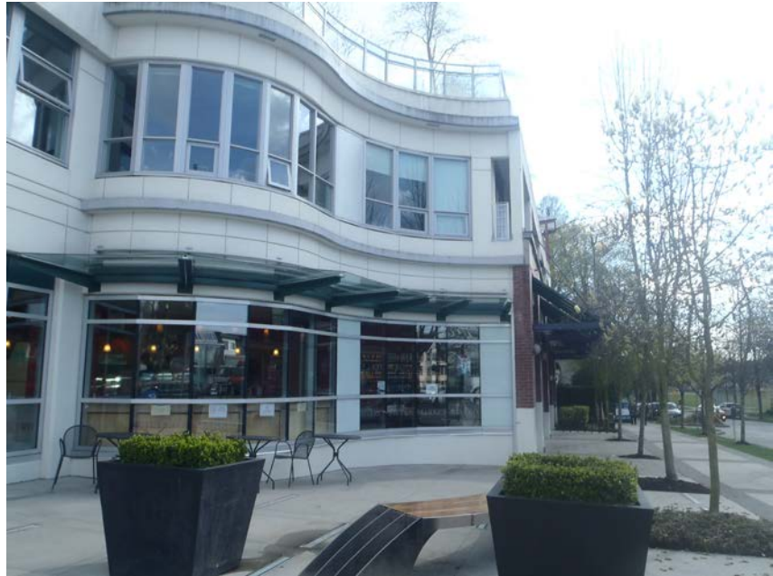
This West Broadway grocery store exceeds the maximum frontage limit, but maintains appeal to pedestrians by providing a public seating area with weather protection along a portion of its frontage (Source: Madeleine Koch)
