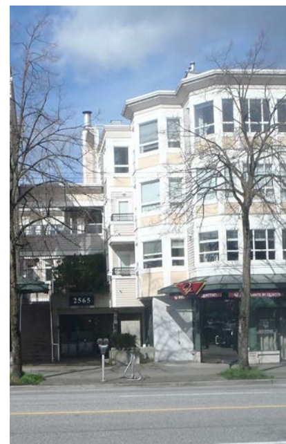
Oriented east to west, this four-storey, mixed-use commercial-residential building enjoys plenty of sunlight (Source: Madeleine Koch)
