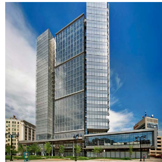
Figure 9. Manitoba Hydro's Hydro Place. Source: www.daniels.utoronto.ca
