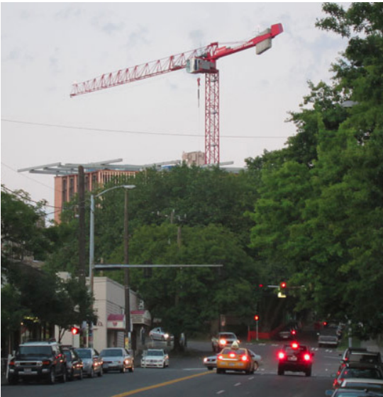
Figure 8. Construction of the Bullit Center. Source: www.citytank.org
