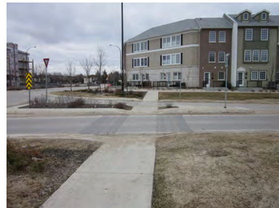
Use of textured pavers, Bridewater Lakes.
