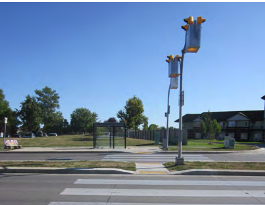
New pedestrian controlled intersection, Dakota Street.
