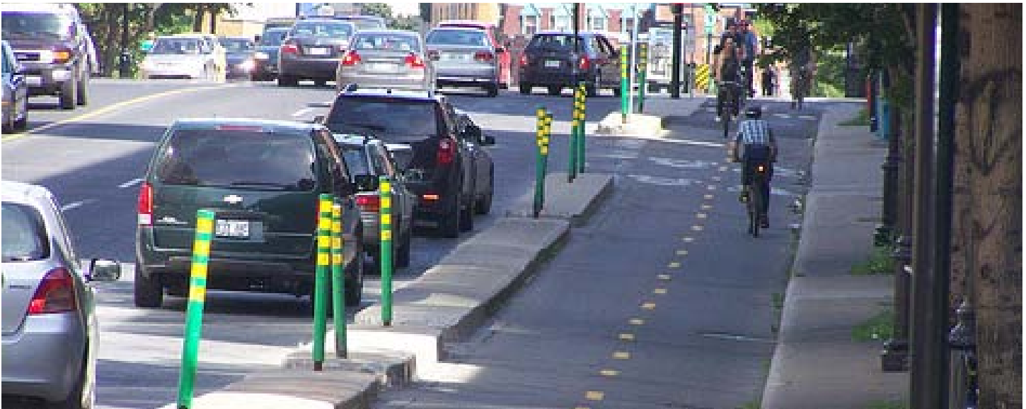
Figure 1: An example of a proper cycle track
