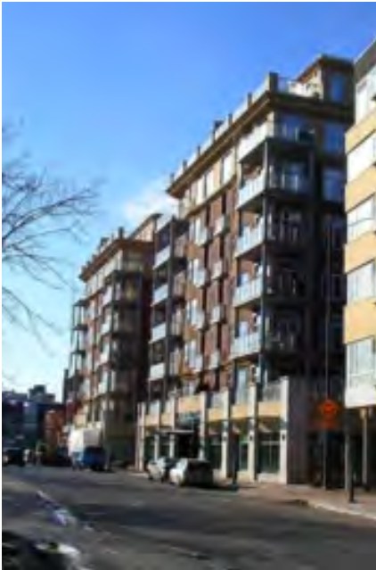
A snapshot of mixed use development on Waterfront drive. (Image Credit: Bridgman Collaborative & McKay Finnigan and Associates, 2008).
