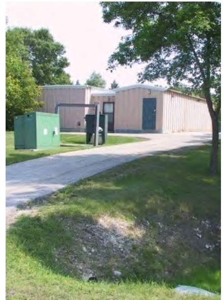
Figure 6: pumping and water treatment station
