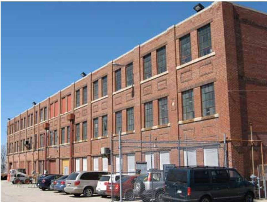
Above: the location of the new Social Enterprise Centre. Current tenants include BUILD, LITE, Social Purchasing Portal, Point Douglas Residents Committee, ACT Mount Carmel Clinic, and Manitoba Green Retrofit. The top floor contains studio space for community artists. (Photo: Jonathan Hildebrand).
