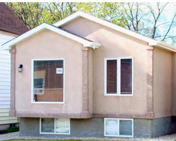
Newly constructed 164 Perth Ave.
