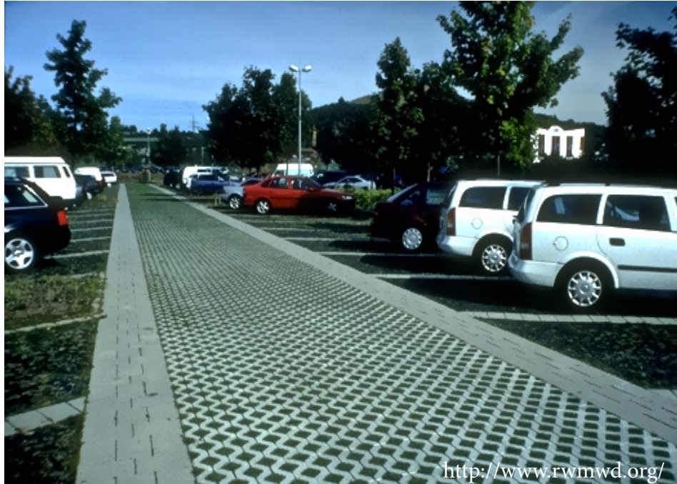
A green parking lot with pervious pavement
