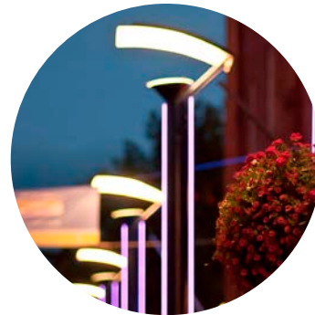
Figure 32: Example of pedestrian street lighting
