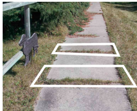
Figure 19: Sidewalks are not in optimal condition - breaks and cracks are highlighted here
