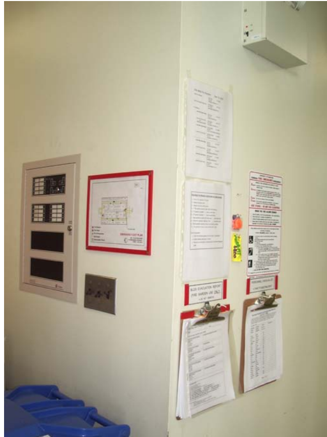
Main Fire Warden Station
