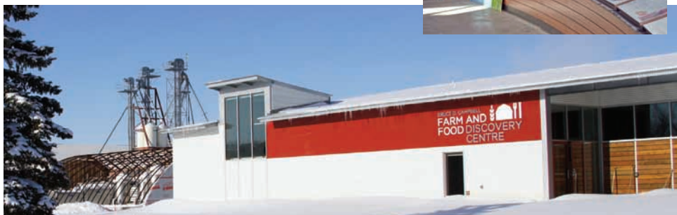
The new Farm & Food Discovery Centre features a number of highlights, including windows into the swine barn (top photo), a fully functional demonstration kitchen (second from top) and hands-on exhibits throughout the centre.
