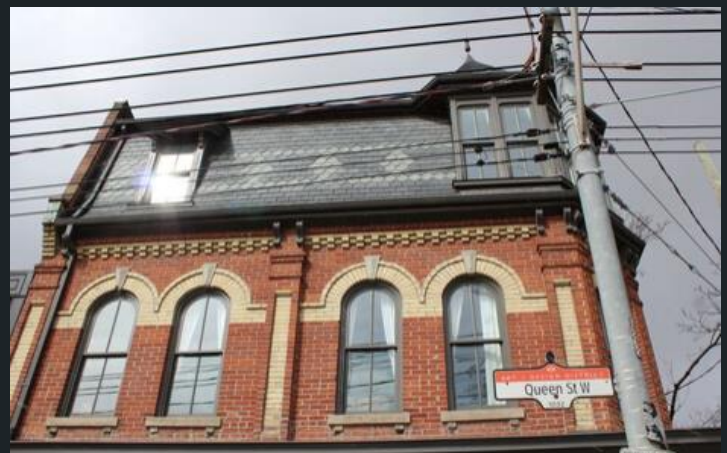
Figure 14: Windows in QSW have a vertical orientation, a 3-dimensional component (are recessed in the wall), and use decorative frame elements. (Source: Pinterest)
