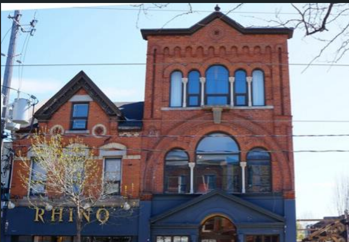
Figure 11: Cornices are employed to add definitions to buildings and to add a level of architectural interest when the building meets the sky. As a horizontal projection, they often cast a shadow, which adds a dynamic effect to the building. (Source: Sunnyside Historical Society)
