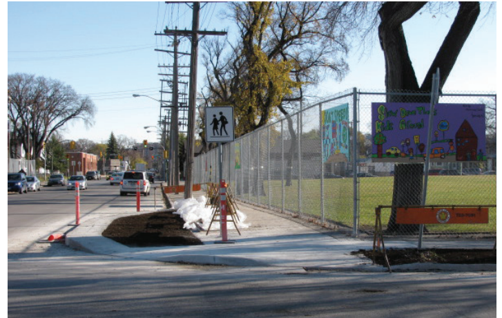
St Matthews Ave and Banning Street bulb-out with student designed safety murals on the fence.
