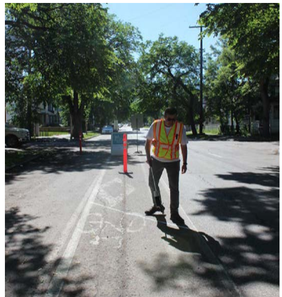
City staff sets up the pop-up bike lanes with spray chalk (Source: City of Winnipeg, 2017b).
