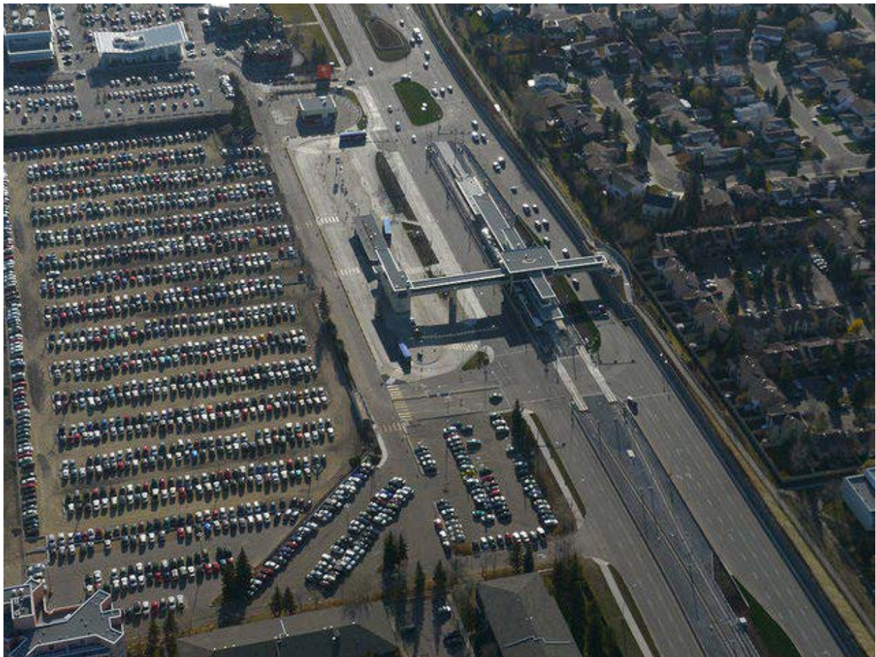
Image 3: Century Park Station and Park-and-Ride. (City of Edmonton, 2011)
