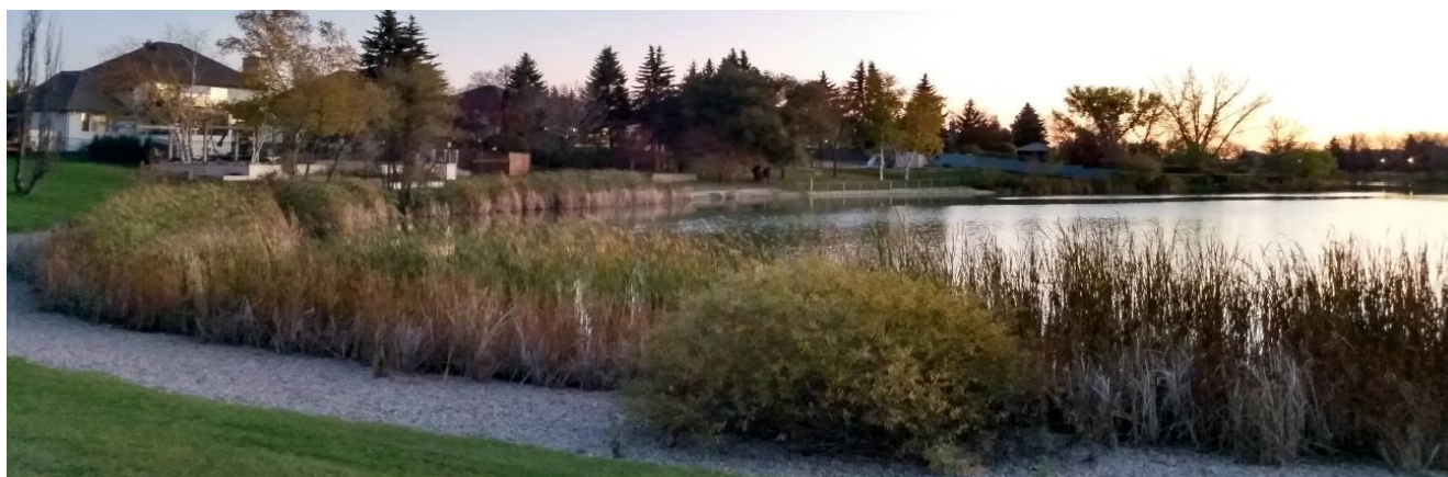
Figure 7: Note the aggregate revetment at the shore edge and reed planting at the retention pond at Linden woods
